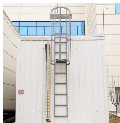
Store purified reuse water temporarily in back discharge tank
